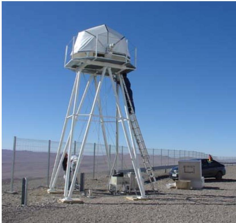
**Figure 4: tensing wires are added to increase the stiffness**
