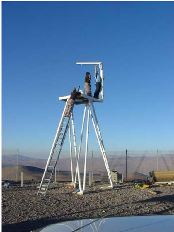
**Figure 2: dome and mount are lifted by means of a removable crane**
