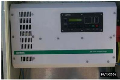
Solar plant charge controller and inverter
