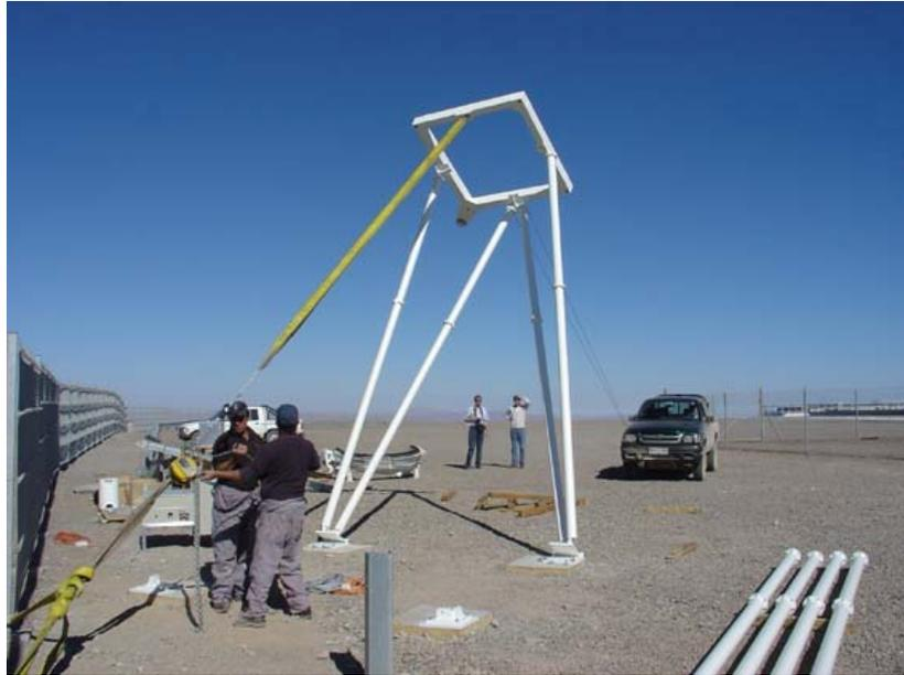
**Figure 1: The tower can be erected without need of a crane**
